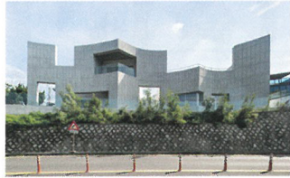
HYUNJOON YOO ARCHITECTS - Wind Fence
